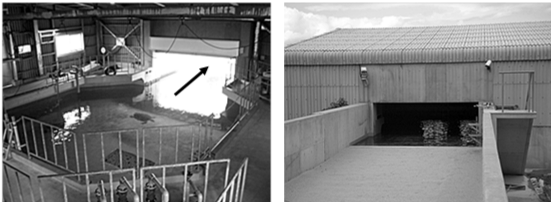
Fig. 2 Photographs of the 250 kL rearing tank (left) and the artificial sandy beach (right). A black arrow shows directions from the 250 kL rearing tank to the artificial sandy beach. The tank and the beach are connected by a gradual slope under the rearing water level so that the female turtles can come up onto the beach for nesting.
