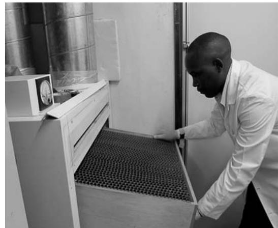
Fig. 10. Lab staff removing used-up intermediate filters
