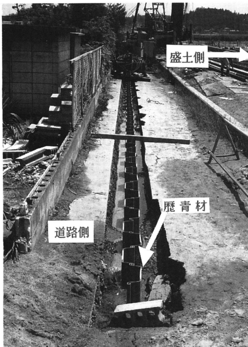
Photo. 1 Situation of SL steel sheet pile installed.
