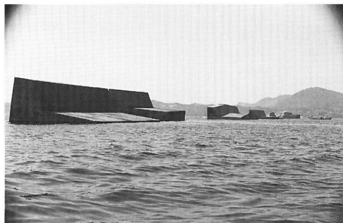
Fig. 3 Photo of damaged breakwater
