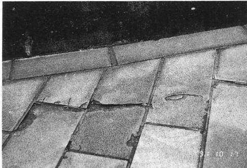
Fig. 3 Situation of settled damage.
