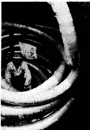
Fig. 17 The equipment of rewinding pipe line
