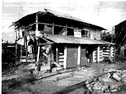
第8図 Damaged house near the Kuwakata coast
