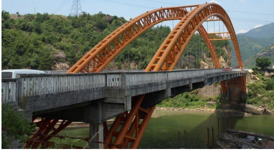
Fig. 1.1 CFST trussed arch bridge
