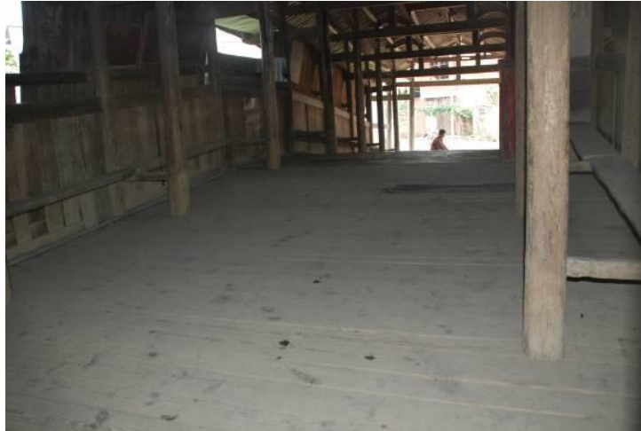
Fig. 4-6 Deck pavement of Xi'nan Bridge
