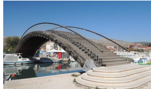
(b) Timber rib arch bridge in Croatia
