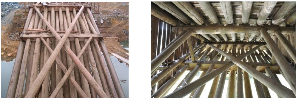
Fig. 2-21 X-bracings
