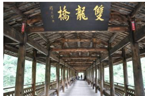
(b) Entrance of the bridge
