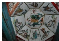
(b) Feiyun Bridge
