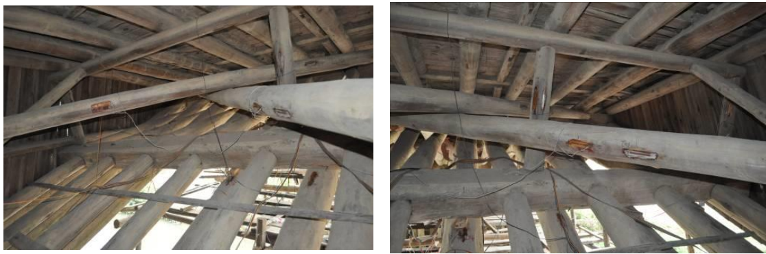
Fig. 4-5 X-bracing and spandrel structure
