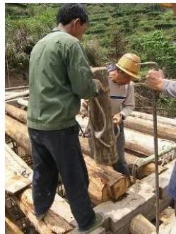
Fig. 2-35 Installation of crown members [12]
