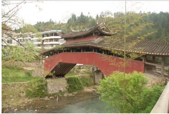
(a) Xidong Bridge
