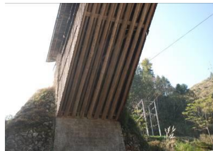
(b) Stone abutment
