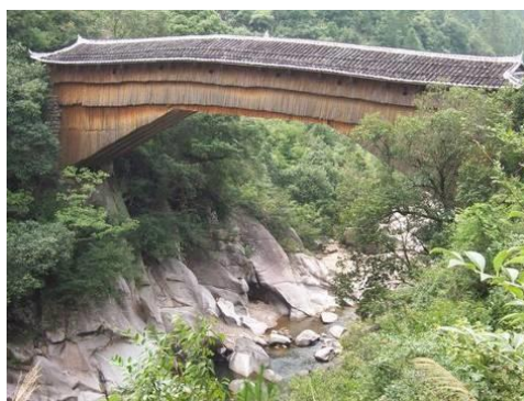
Fig. 3-4 Quondam Baixiang Bridge
