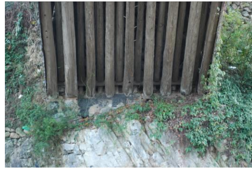
(b) Fushou Bridge
