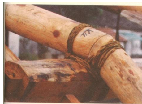
Fig. 2-14 Binding of Bianhe Rainbow Bridge
