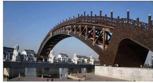
(b) Xujiang Bridge in China
