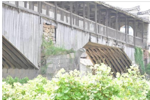
Fig. 2-17 Abutment of Yuqing Bridge
