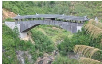
(b) Reconstructed Jinzao Bridge
