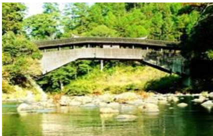
(a) Quondam Jinzao Bridge
