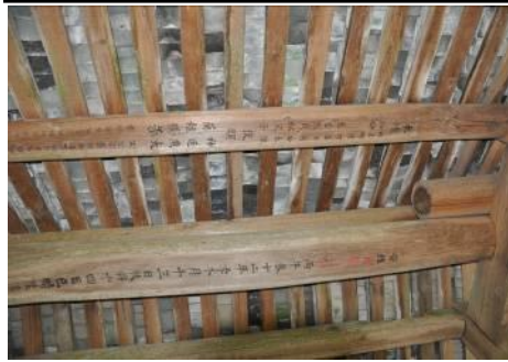
Fig. 2-40 Ridges of the covered house
