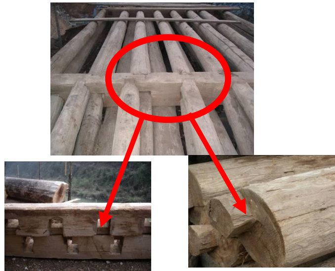
Fig. 2-19 Mortise and tenon nodes
