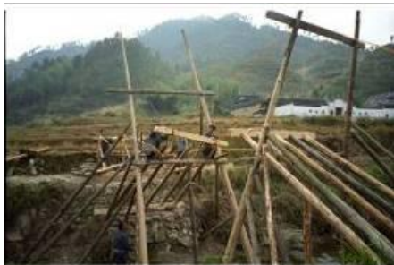
Fig. 2-33 Installation of transversal beam [12]
