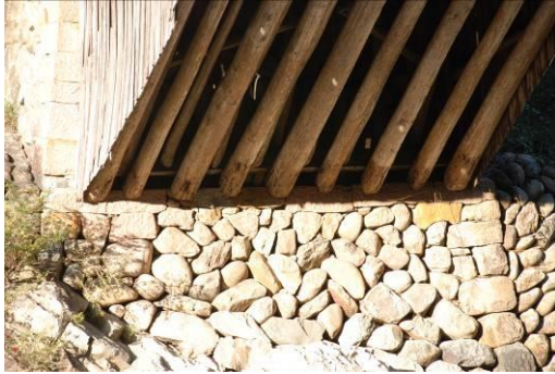
(c) Hongjun Bridge
