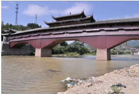
(c) Buliang Bridge
