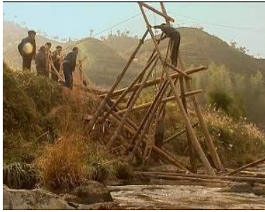
Fig. 2-31 Lifting arch ring members
