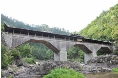
(a) Shuanglong Bridge General view
