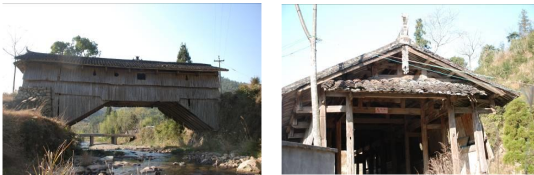
Fig. 2-58 Overhanging gable roof
