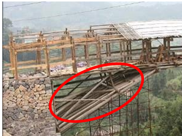
Fig. 2-22 Spandrel structure (called as Horse leg in folk of China)
