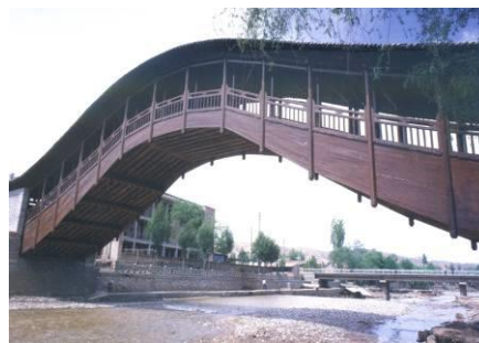
Fig. 2-1 Baling Bridge in Gansu Province
