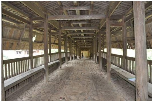
(c) Jielong Bridge
