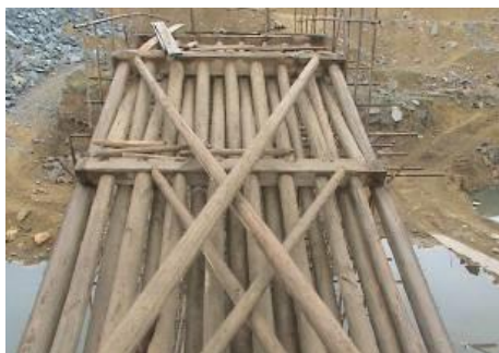
Fig. 2-37 X-bracings [12]
