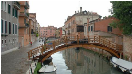
(a) Timber rib arch bridge in Italy
