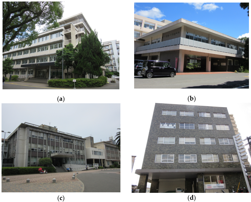
Figure 2. External views of the four office buildings surveyed in this study: (a) B1, (b) B2, (c) B3, and (d) B4.
