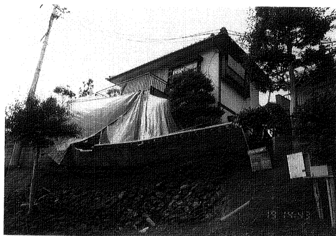
Photo 2. Collapse of a concrete block wall at the top of the landslide (Photo July, 1, 1997).
