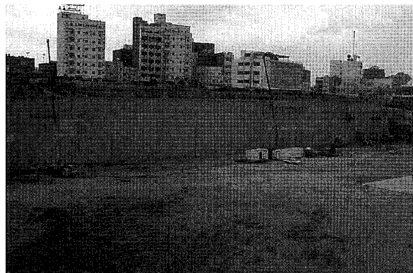
Photo 3 Diaphragm wall after construction.
