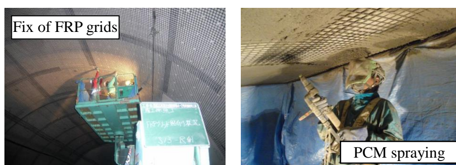
Fig. 2.8 Fiber reinforcement method (Higashi et al., 2012).
