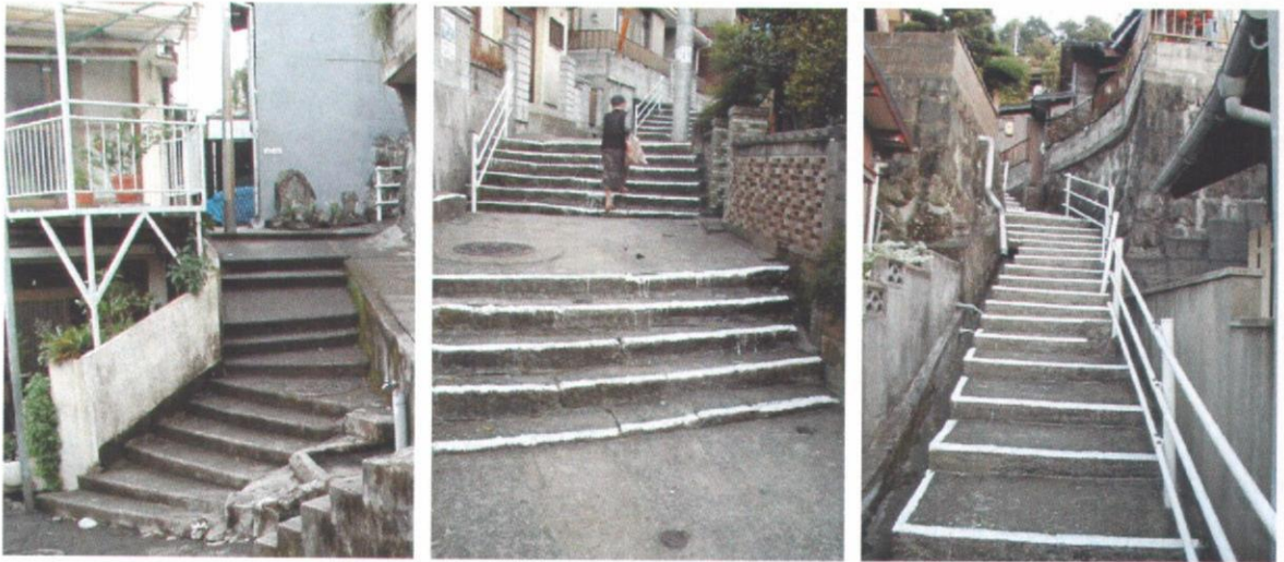
(a) highly irregular stairs
