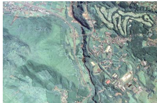
Fig. 6(b) Bird's eye view of Aso Big Bridge and the original Tatsuno hill from GIAJ (2013).
