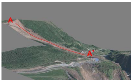
Fig. 11(b) Landslide profile of the Tatsuno hill.
