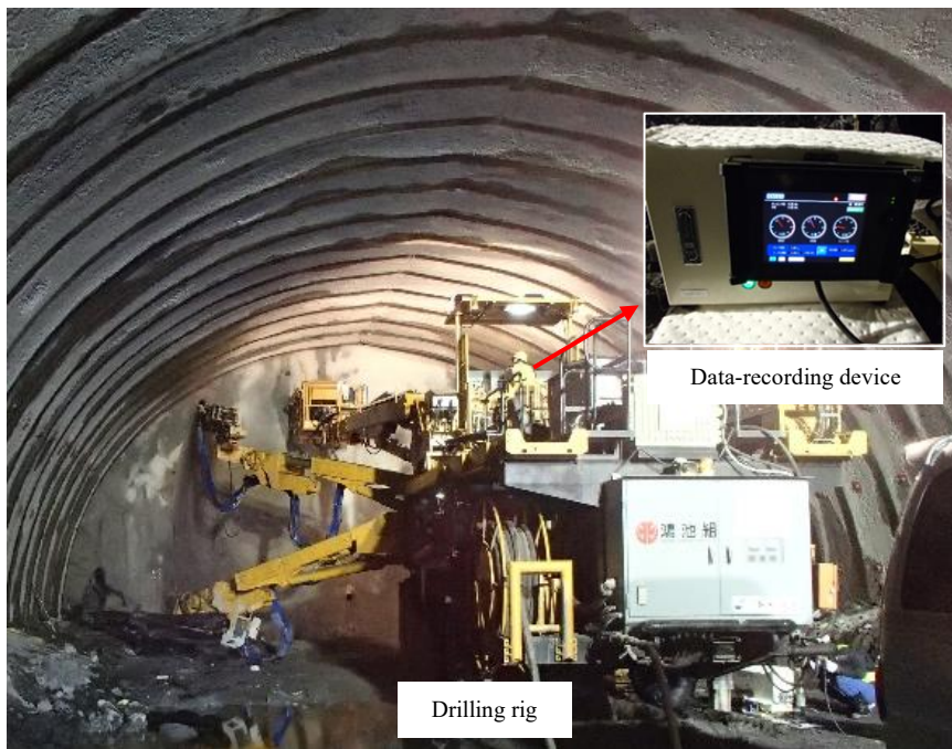
Fig. 2.6 The hydraulic rotary percussion drill
