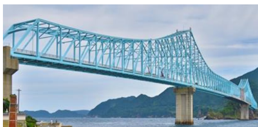
(a) Truss bridge
