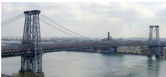
(c) Suspension bridge
