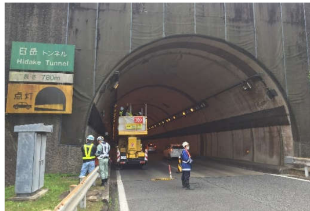
Fig. 8 The Hidake Tunnel in Japan
