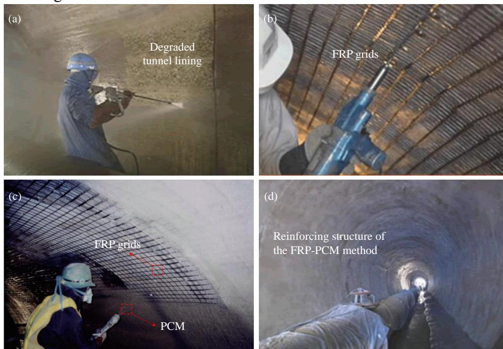
**Fig. 4.1** Application of the FRP-PCM method on degraded tunnel linings (FPR Grid Method Association of Japan): (a) surface treatment; (b) fix the FRP grids; (c) spray the PCM; (d) after the construction.
