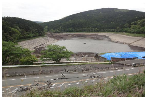
(c) Damage to surrounding roads
