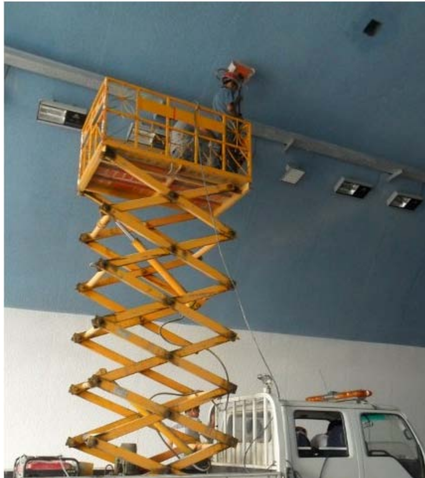
Fig. 2.8 An example of data collection of GPR.
