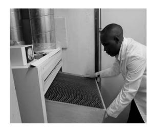
Fig. 10. Lab staff removing used-up intermediate filters
