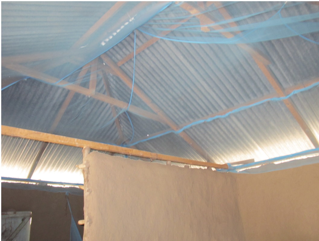
Fig. 1. Intervention with the permethrin-impregnated ceiling net.
