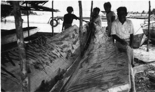
Fig. 10. House boat being built in a shed at Bakori I.
